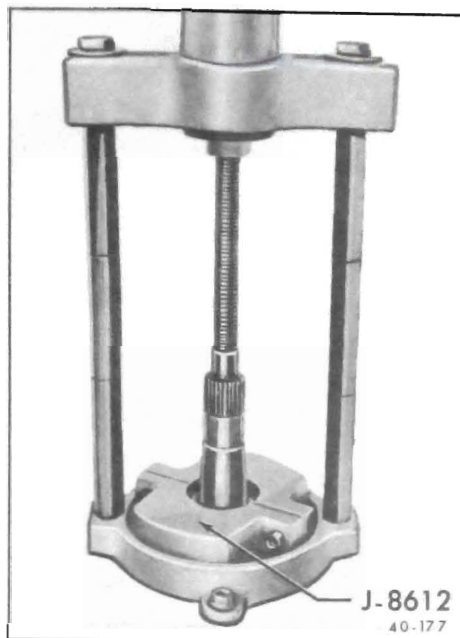
Figure 40-189 - Removing Rear Pinion Bearing
