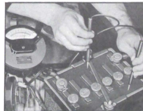
Figure 10-3—Light Load Test
